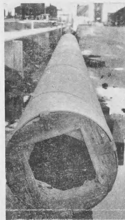
Looking down the barrel of a cannon! Here are several sections of the "Big Inch" lying on the ground near the paint shop. 4000 feet of this big pipe will be installed this month.
